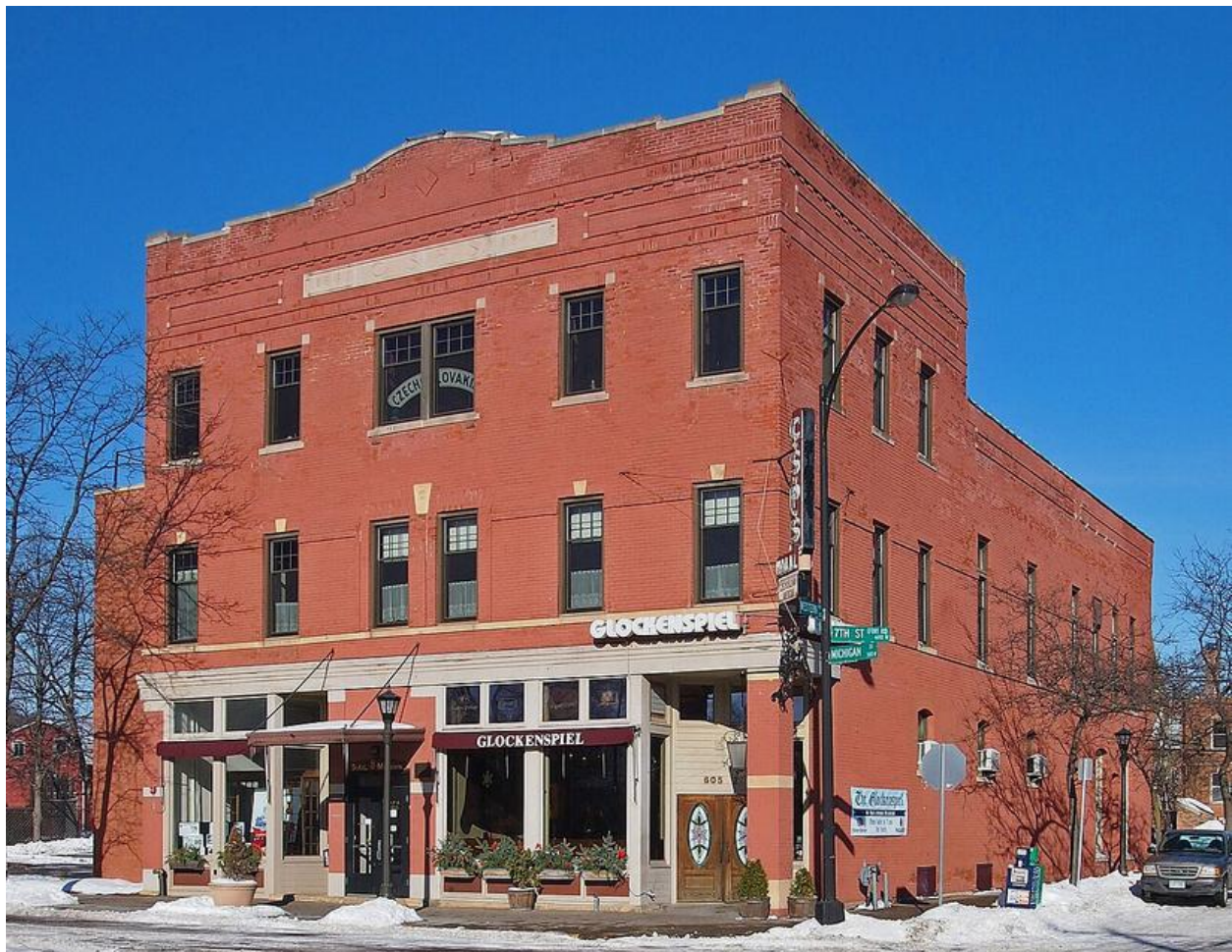
C.S.P.S. Hall, also known as Czech Hall or as CSPS Sokol Hall. 383 W Michigan St, St Paul, MN 55102.
